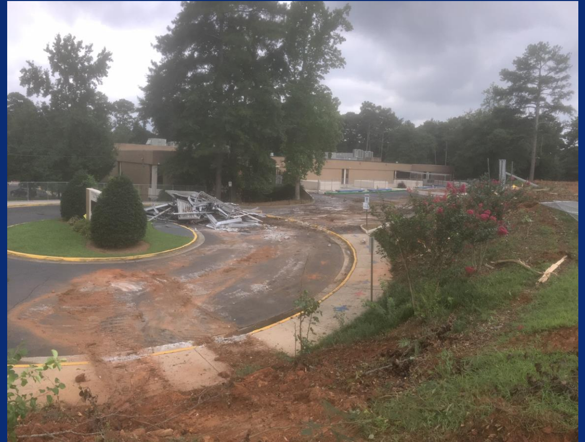
East Side Existing School Canopy & Richland Loop Demolition
